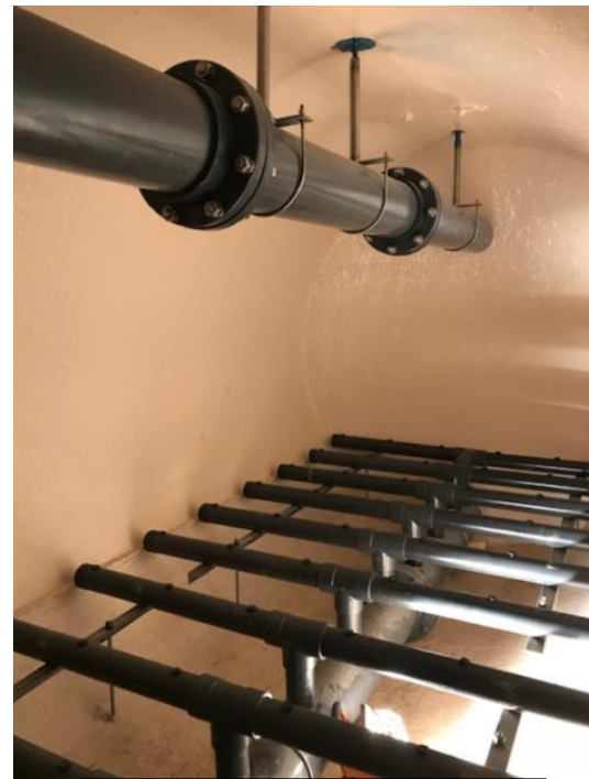
Fig.2 Post-Rehab Before Sand Valve Installation and concrete fill
