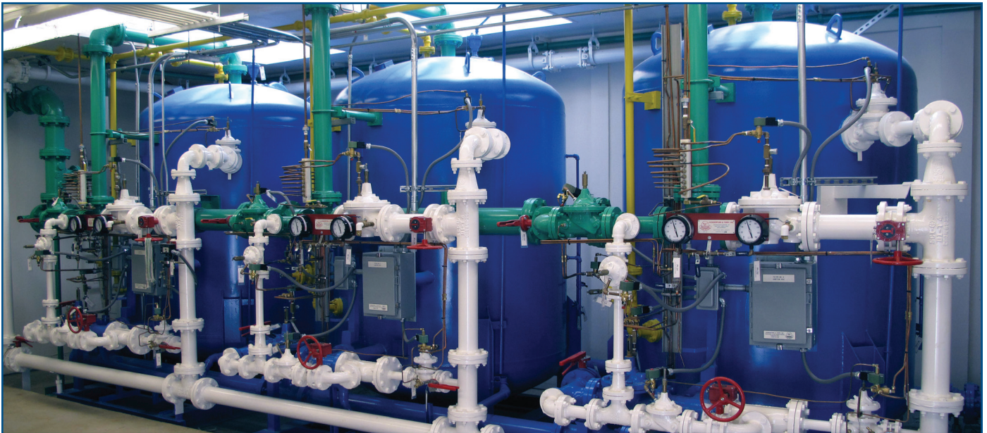
This is an example of the 1.5 MGD municipal filter installation with air/water wash, by Hungerford & Terry.
