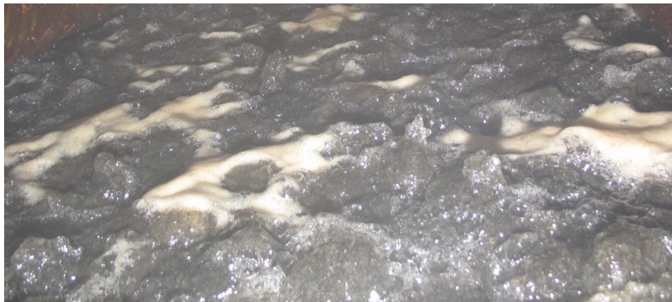
Horizontal Filter media in Air Scour mode
