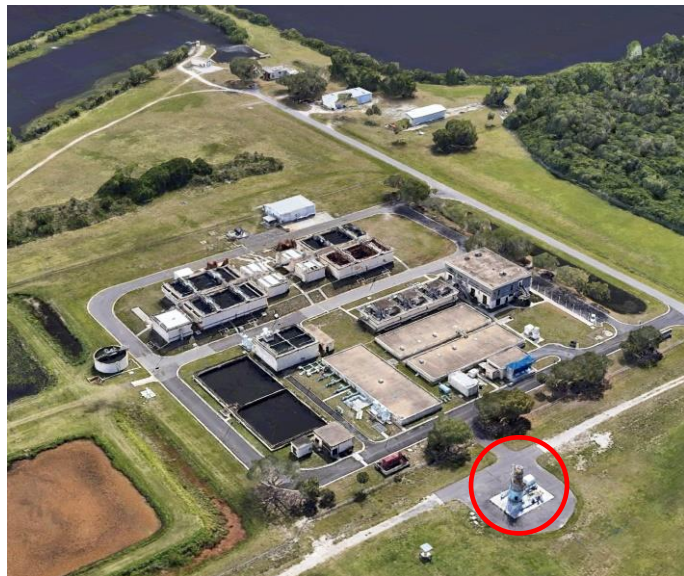
WTP & Operational ASR2
