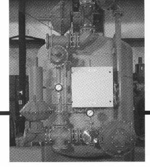
Hungerford & Terry, Inc. is also a licensee of the Dowex Upcore<sup>®</sup> packed-bed ion exchange system. This technology offers all of the advantages of a counter-current regenerated system plus offers greater capacity and reduced waste volumes by making the most efficient use of the vessel size. This system also lends itself to retrofitting existing systems so that old, inefficient demineralizers can benefit from this technology at a fraction of the cost of a new system of equal performance.
