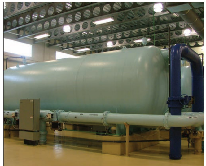
Hungerford & Terry, Inc., Clayton, NJ - pretreatment units shown above consist of three GreensandPlus™ pressure filters. Anthracite and GreensandPlus media are used to remove iron and manganese in order to protect the RO membranes.
