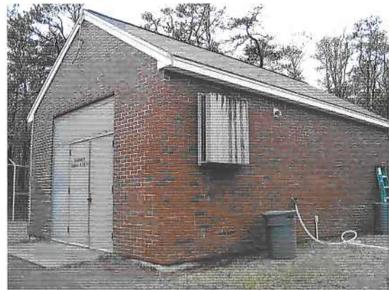
FIGURE 3-2 CORROSION CONTROL FACILITY
