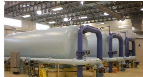
Hungerford & Terry, Inc., Clayton, NJ – pretreatment units shown above consist of three GreensandPlus™ pressure filters. Anthracite and GreensandPlus media are used to remove iron and manganese in order to protect the RO membranes.
