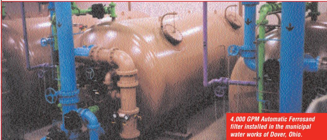
**4,000 GPM Automatic Ferrosand filter installed in the municipal water works of Dover, Ohio.**
