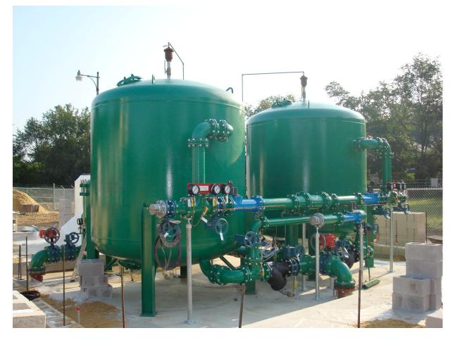
Clayton, NJ - Hungerford & Terry, Inc. was selected by the City of Vineland, New Jersey to design and supply equipment to remove radium from four municipal city wells during 2009 and 2010. All of the systems for the four designated wells are identical in specifications and design and each one includes two 102" diameter (2.5909m) exchangers to remove radium.
